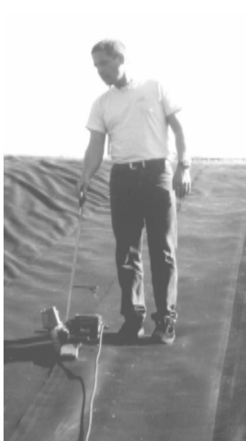
Thermobond dual track seams that can be tested using air pressure.
