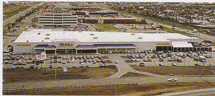
Eagle Hardware, Edmonton, Alberta Mechanically Fastened Hi-Tuff Roof System
