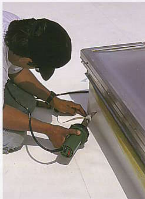
Hot-air corner fabrication with a hot-air hand welder.
